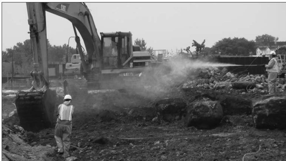
Excavation is the method of choice for cleaning up the Garfield Avenue Site, which PPG has been doing since July as part of the initial cleanup.
